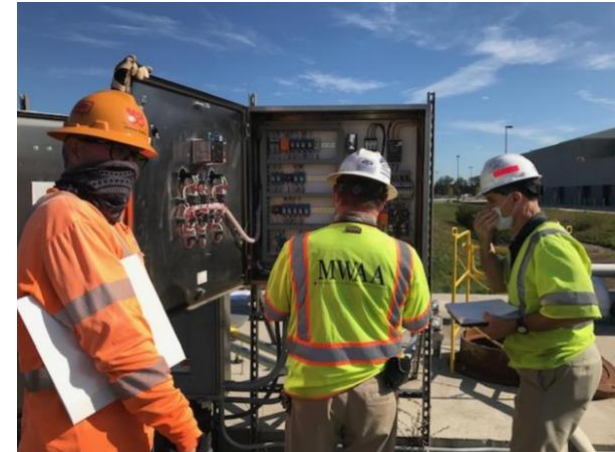
Sanitation lift inspection at the Yard
