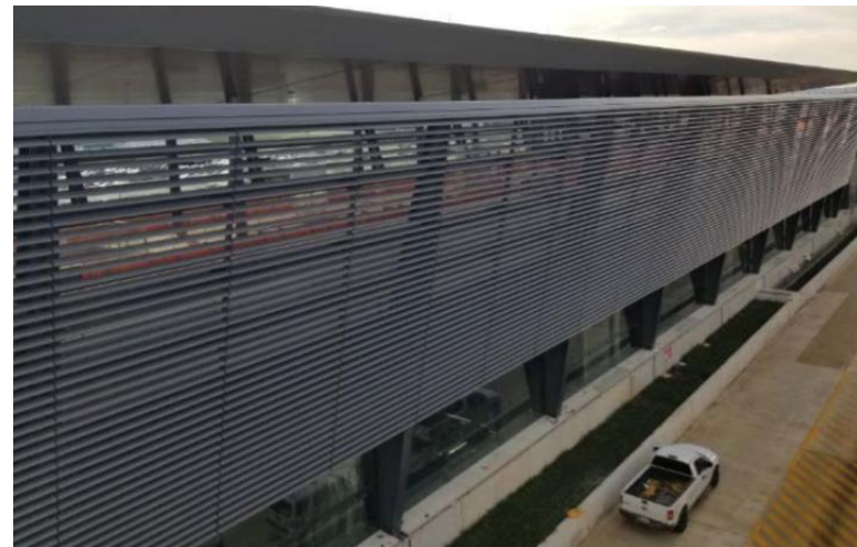
Dulles Station Louvered Screen Wall
