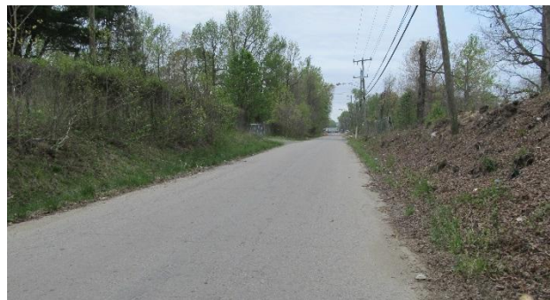
Cinder Bed Road north of Hill Park Drive
