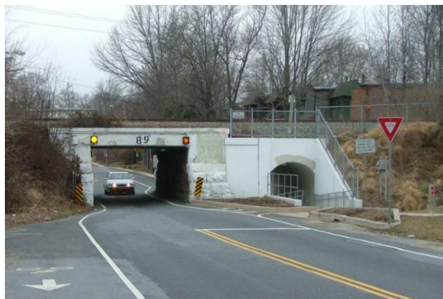
Casho Mill Road Pedestrian Underpass, Newark, Delaware
