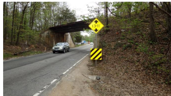
Fort Belvoir Railroad Spur Bridge
