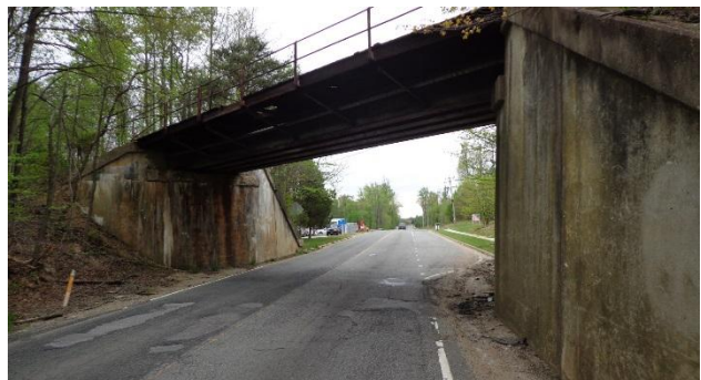
Existing Fort Belvoir Railroad Spur Bridge
