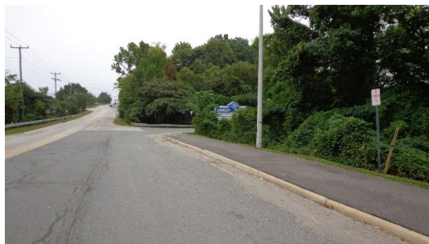
Backlick Road facing east toward Cinder Bed Road
