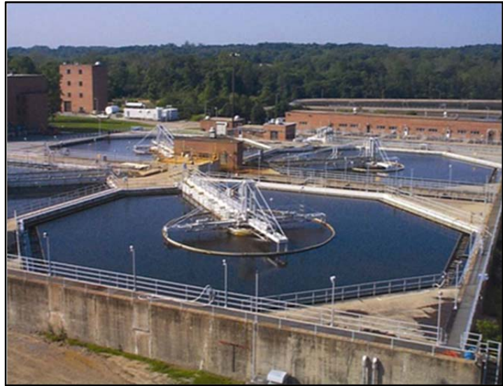
Photo of the Noman M. Cole, Jr. Pollution Control Plant
