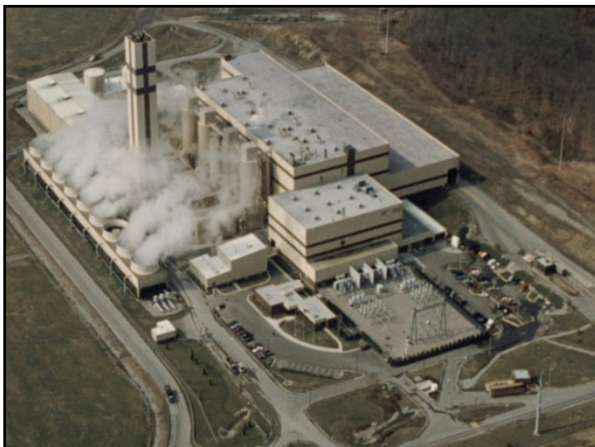
I-95 Energy/Resource Recovery Facility
