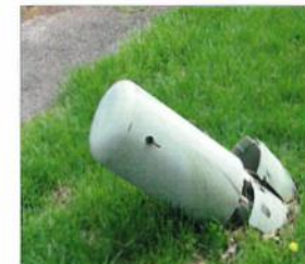
Damaged pedestal
