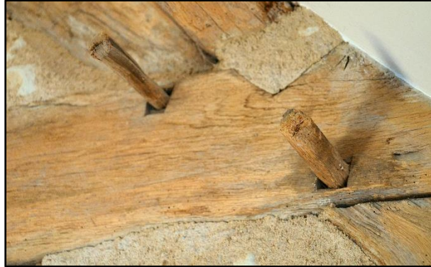
Wooden Pegs used in Joinery, Courtesy of Wikimedia Commons
