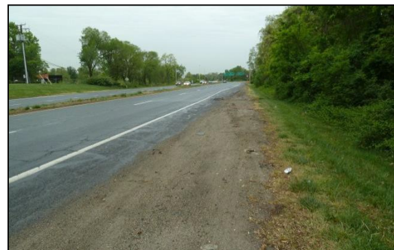
Multilane road with relatively narrow shoulder Source: Toole Design Group.
