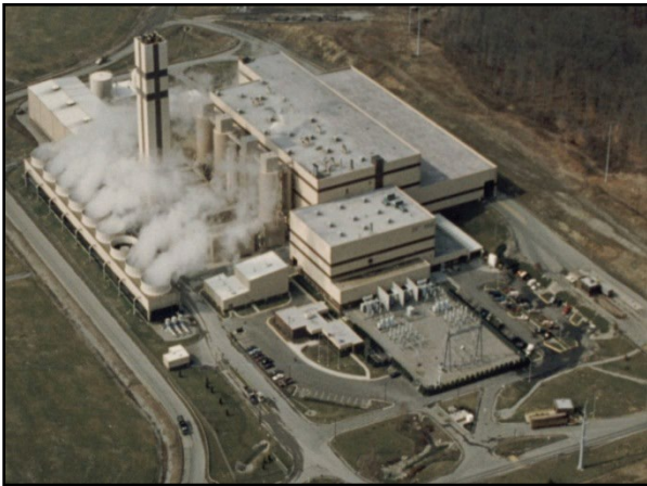
I-95 Energy/Resource Recovery Facility
