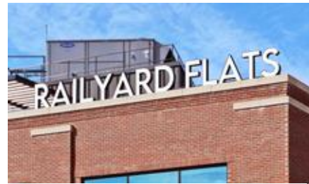
Figure 2: Example of Roof Sign Source: Pride Neon Sign Solutions
