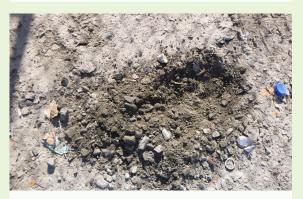
Photo 3 - Surface gravel clogged by excessive sediment.
