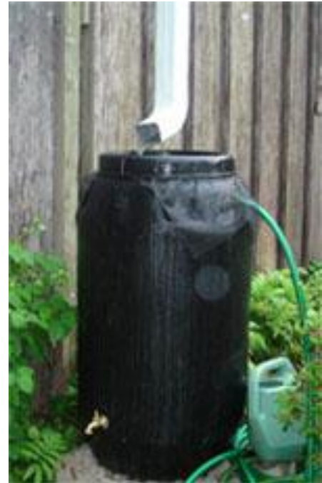
Photo 4.13 Typical Rain Barrel
