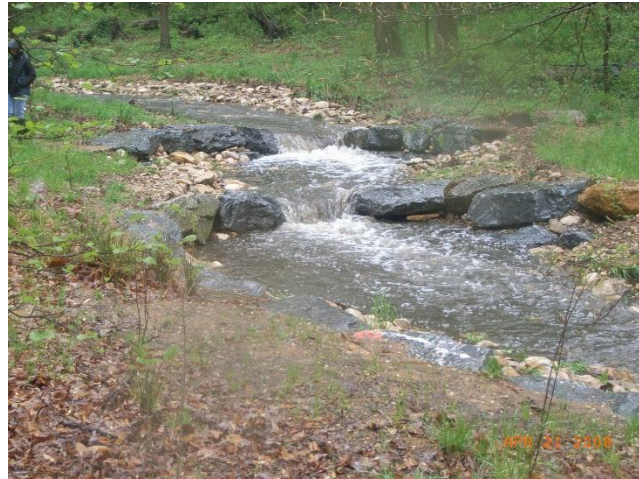
Photo 4.10 Step Pool Channel Source: Arlington County, VA
