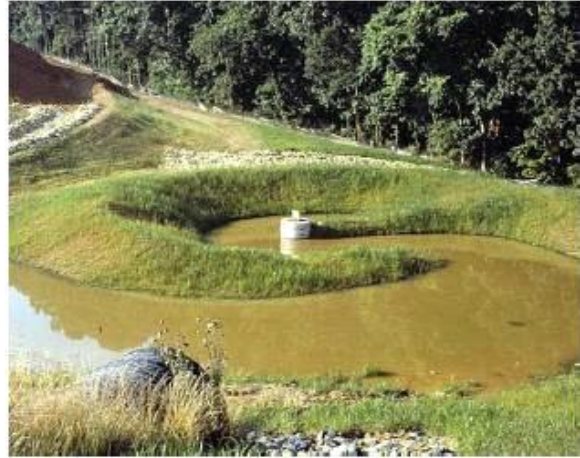
Photo 4.1 Extended Detention Basin Full of Stormwater
