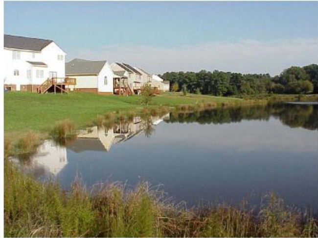
Photo 4.3 Retention Basin Source: Virginia Stormwater Management Handbook
