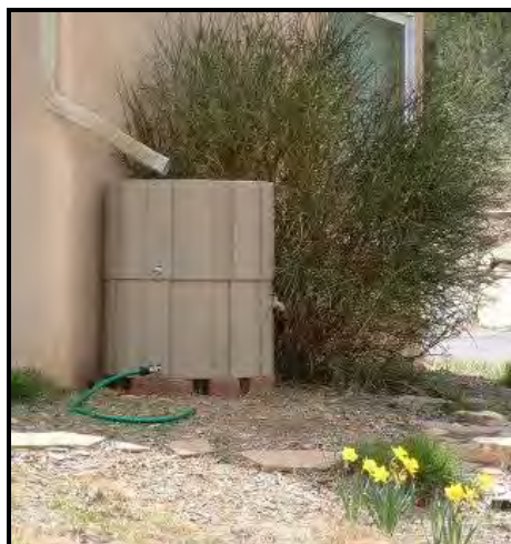
Rain barrel & above-ground cistern (Sources: Prince George's County 1999; www.aridsolutions.com ; and www.plastmo.com )
