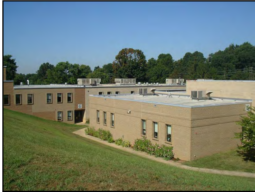
Figure 6-4. Example of a county facility (Shreveewood Elementary School) that could present a good opportunity for a green roof
