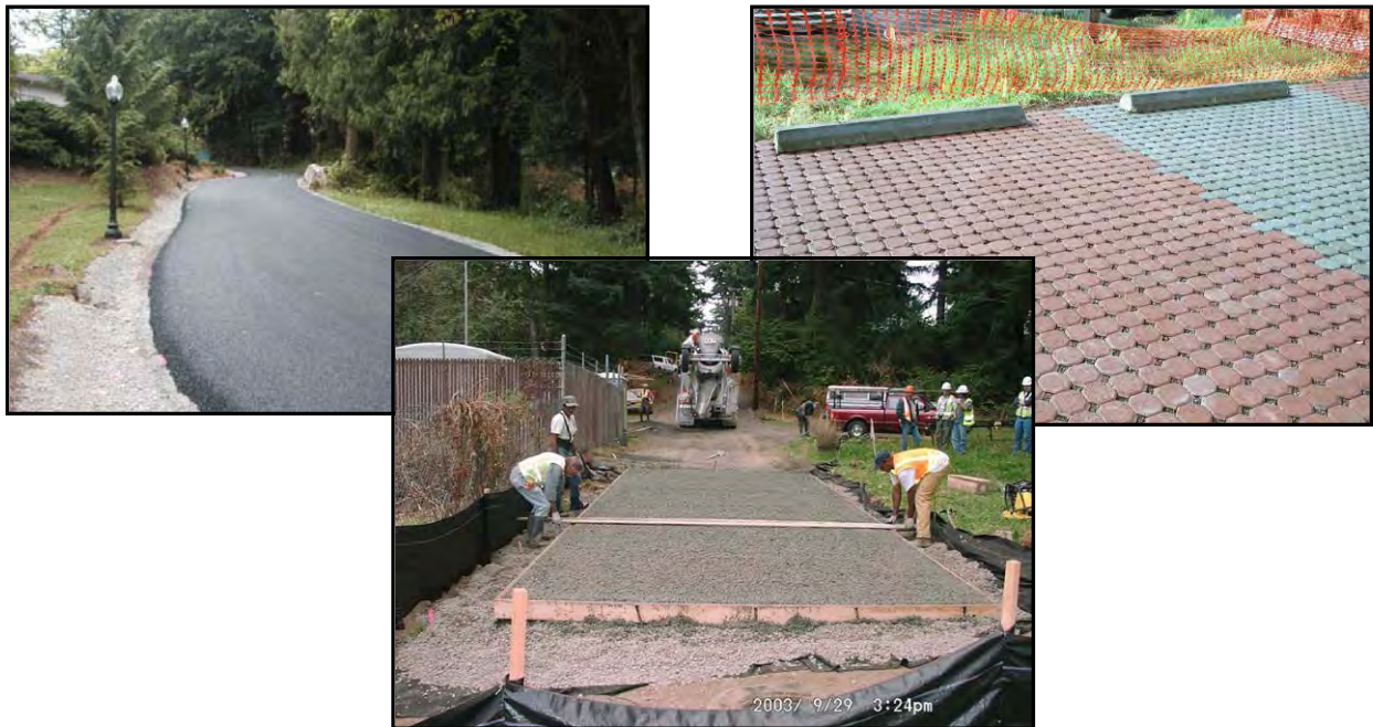
Permeable pavers – asphalt, concrete, and block (Source: City of Portland 2003)
