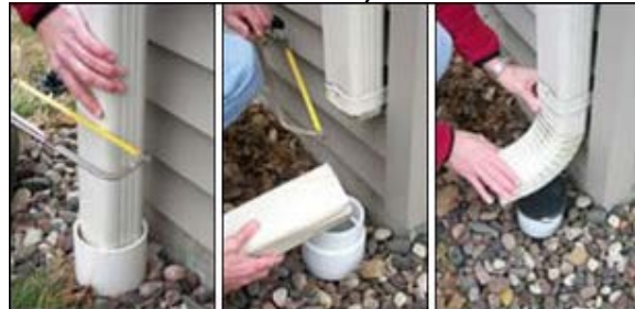
Figure 4-21: Disconnecting a downspout (Source: City of Toronto)
