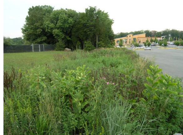
Figure 4-9: Vegetated swale (Source: Fairfax County)
