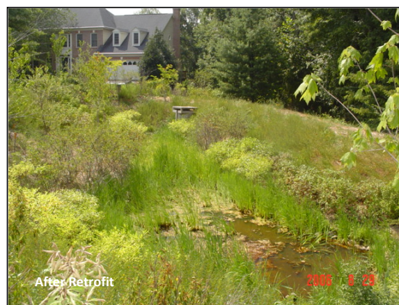
Figure 4-4: Stormwater dry pond retrofit (Source: Fairfax County)
