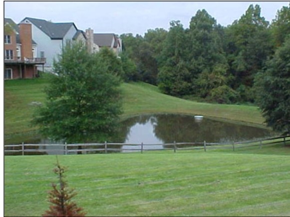
Figure 4-2: Stormwater Management wet pond (Source: Fairfax County)
