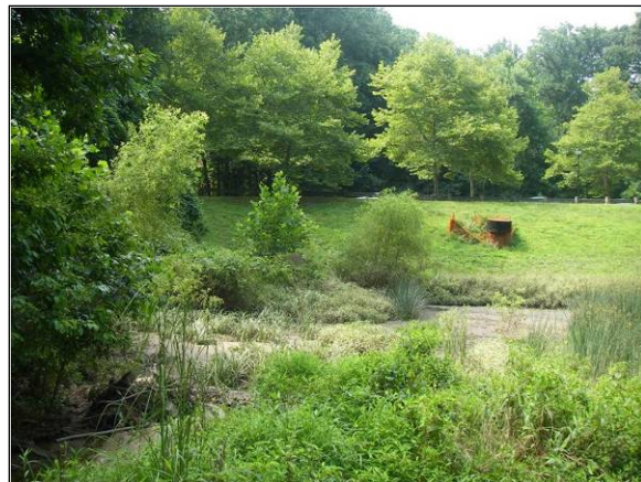
Figure 4-3: Engineered stormwater wetland (Source: Fairfax County)
