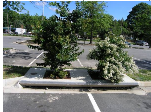
Figure 4-10: Tree box filter (Source: Fairfax County)
