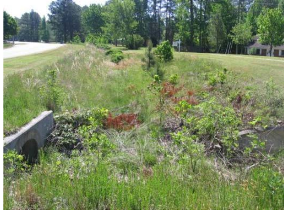
Figure 4-14: Vegetated swale for roadside drainage (Source: KCI)
