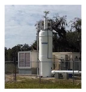
Figure 3-13: Biotrickling filter (courtesy of BioAir Solutions).
