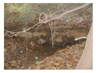
Photo 3.22 Erosion at outfall pipe located near Mill Creek Landing (DFDF003.P001).
