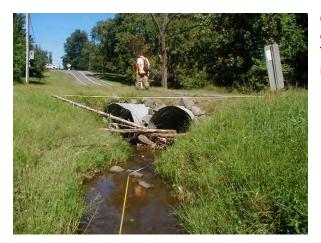
Culvert #17 (Photo 3.132) overtopped for events less frequent than the 5-year storm. This can be classified as a local road, which means the culvert should be able to pass the 10-year event.
