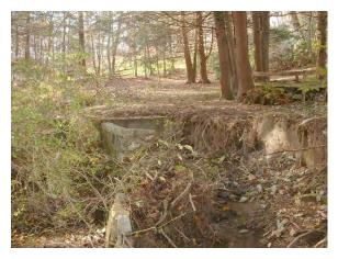
Photo 3.26 Severe erosion that could pose a threat to road safety along Route 7 to the east of Carpers Farm Way (DFCR001.E001).
