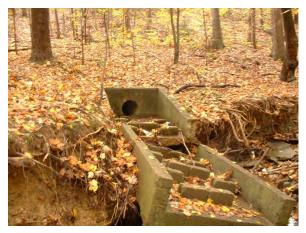
Photo 3.45 Erosion at a 12-inch outfall located just south of North Shore Drive (DFCR013.POO3).
