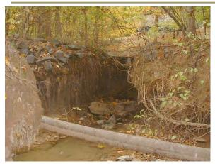
Photo 3.56 An 18-inch outfall causing severe erosion located downstream of the outfall shown in Photo 4.1 (DFSB006.P005).
