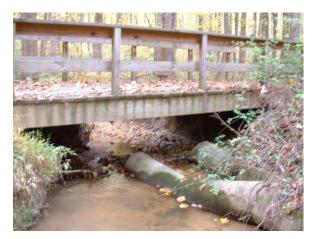
Photo 3.65 Wooden bridge where stream flow is causing moderate erosion. Located just west of Steeplechase Drive (DFGL008.C001).
