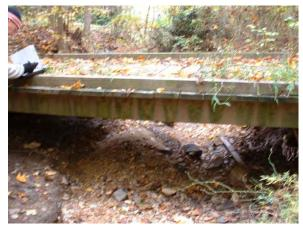
Photo 3.64 Wooden bridge where stream flow is causing moderate erosion. Located just off of Bassett Lane (DFGL008.C004).
