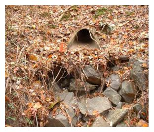
Photo 3.2 Erosion below stormwater pipe located at the end of Milburn Street (DFCH021.P001).
