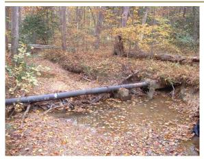
Photo 3.60 Exposed sanitary utility line crossing stream (DFSB006.U002).
