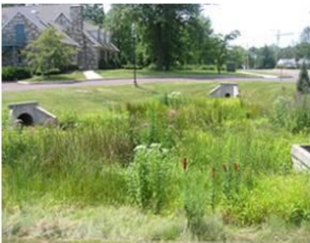
Figure 4-1: Dry stormwater pond
