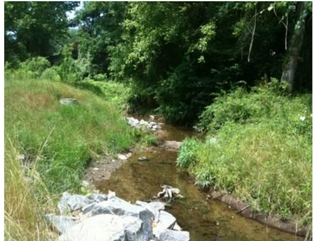
Figure 4-8: Stabilized stream banks
