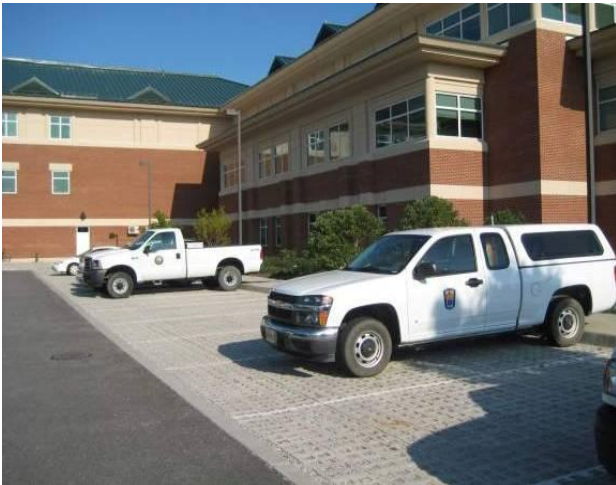
Figure 4-3: Parking lot pervious pavement
