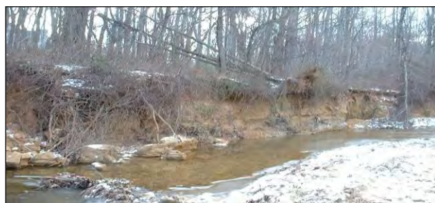
Severe erosion was observed at Scotts Run north of Old Dominion Drive
