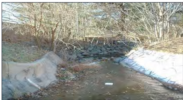
Concrete lined portion of Dead Run
