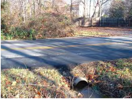
Photo 3.4 A culvert (PHPH036.C002) at Popes Head Road has a minor impact on the stream
