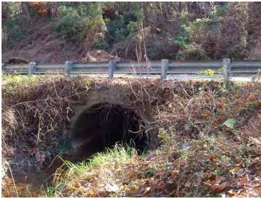
Photo 3.6 A culvert (PHPH028.C002) at Fairfax Station Road has a minor impact on the stream
