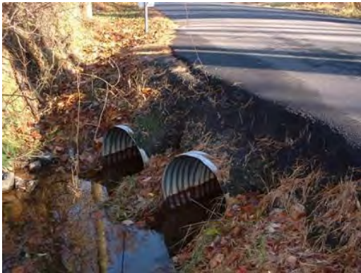
Photo 3.10 A double culvert (PHCC006.C001) at Newman Road has a minor impact on the stream
