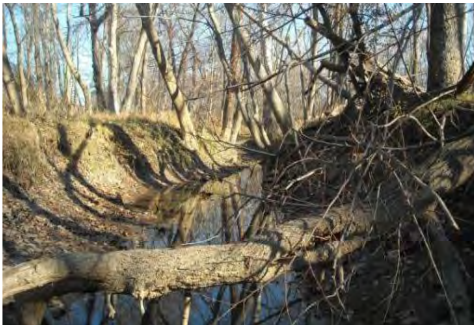
Figure 1: Deeply incised channel with severe erosion
