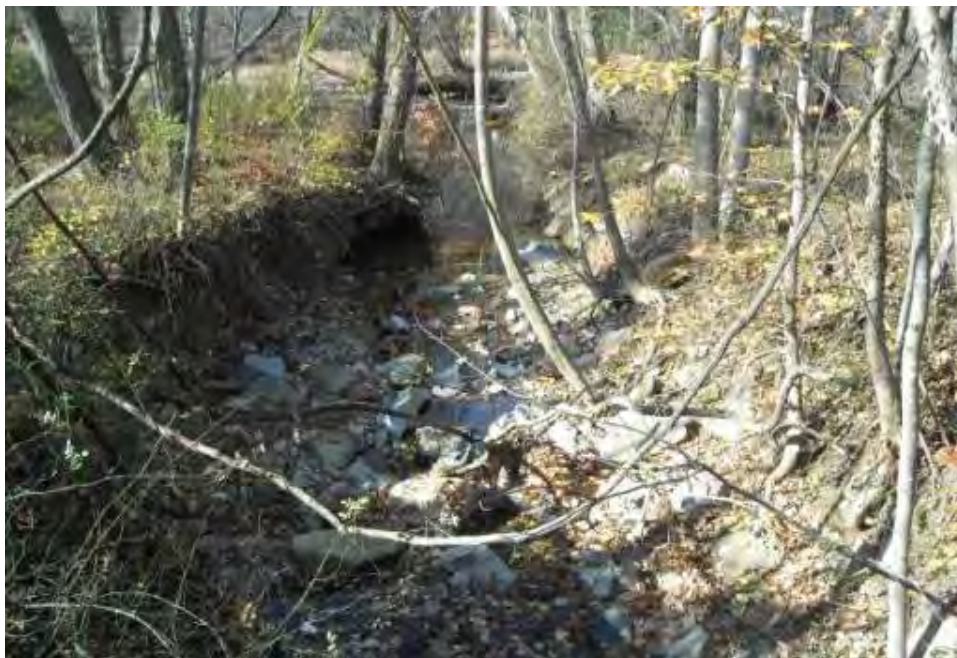
Figure 1: Incised channel with severe bank erosion
