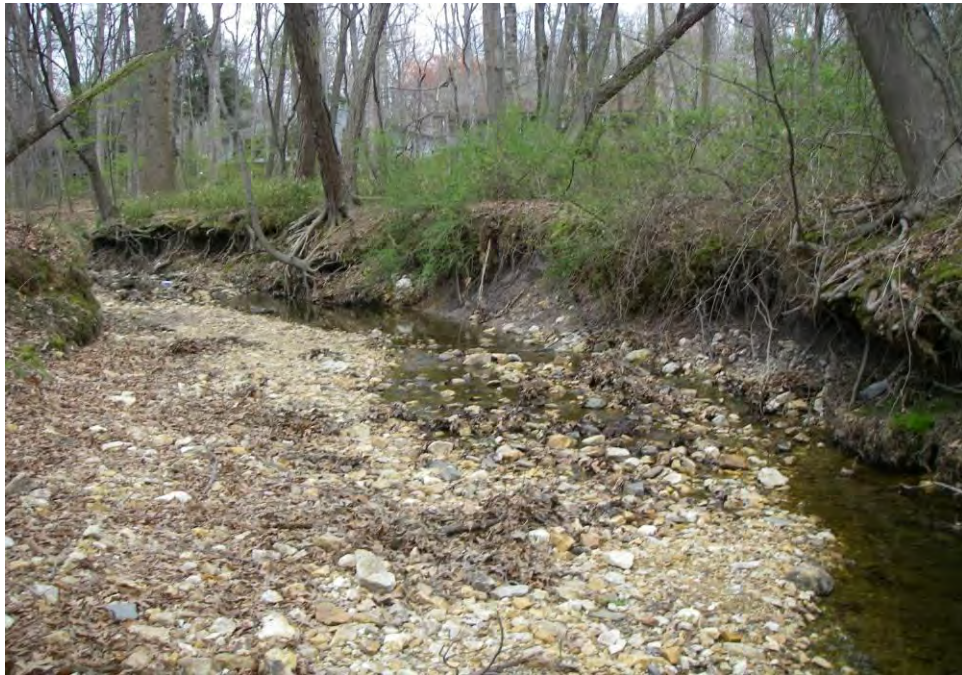
Site Photo: Incised and over-widened channel with moderate bank erosion
