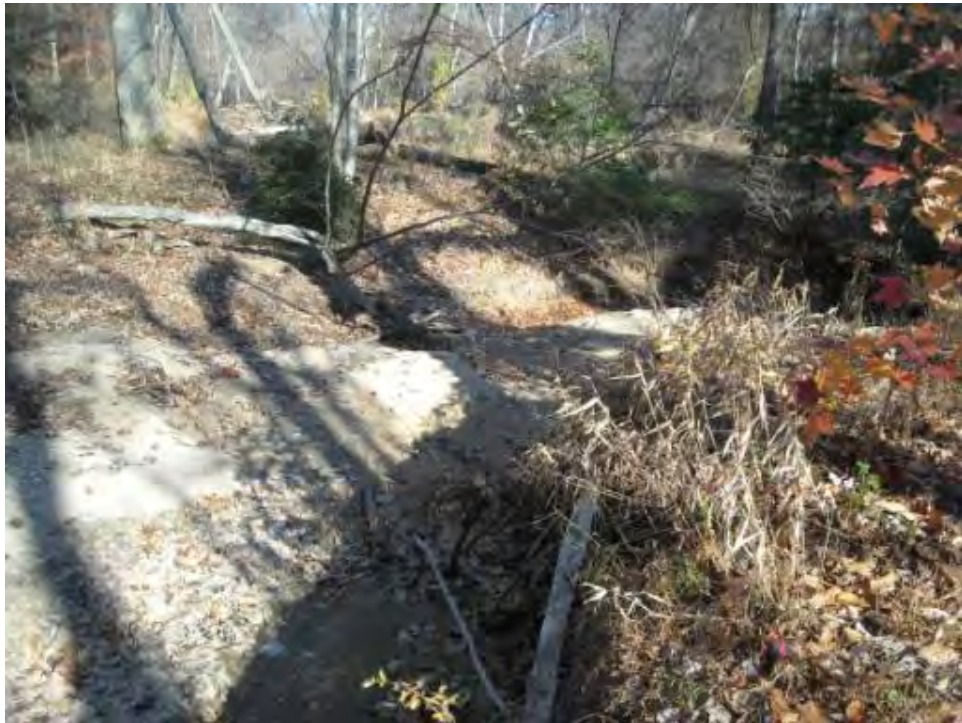
Figure 2: Overflow channel with large sand deposits
