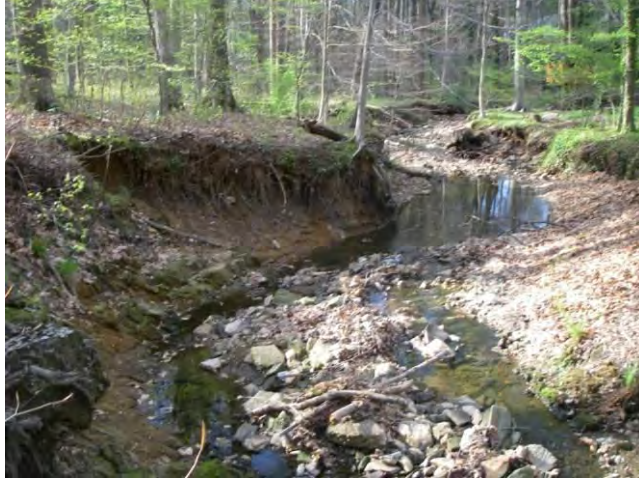
Site Photo: Moderate erosion on meander banks
