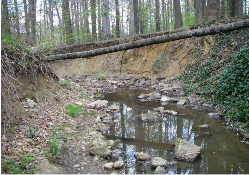
Site Photo: Incised channel with severe meander bend erosion
