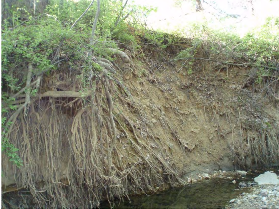
Figure 1: Eroded banks along Highland Street
