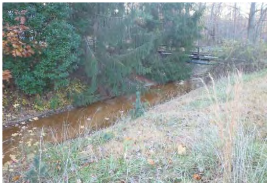
Figure 1: Existing concrete lined stream channel with private driveway bridge
