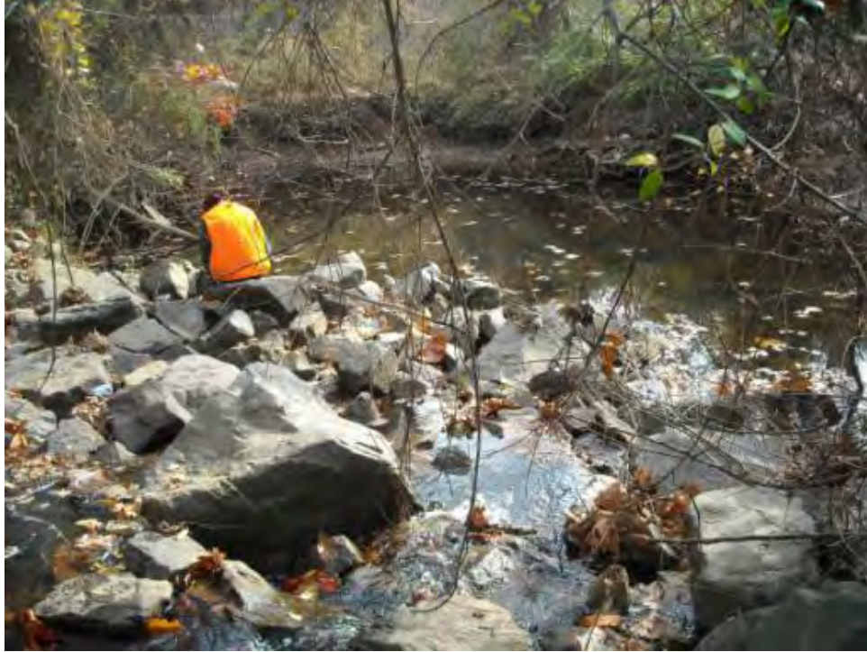
Figure 1: Severe bed and bank erosion just downstream of a utility covered by riprap near the confluence with Accotink Creek
