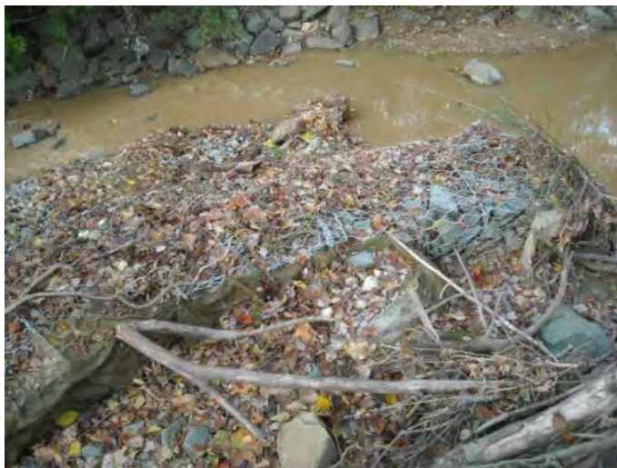
Figure 2: Existing gabion baskets within the channel
