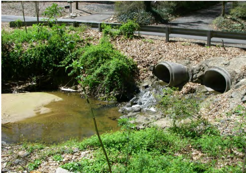
Site Photo: Downstream side of culvert under Woodlark Drive
