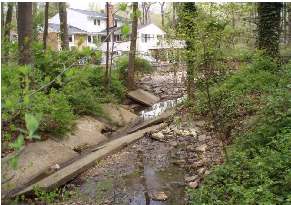
Site Photo: Concrete/rip rap in downstream portion
