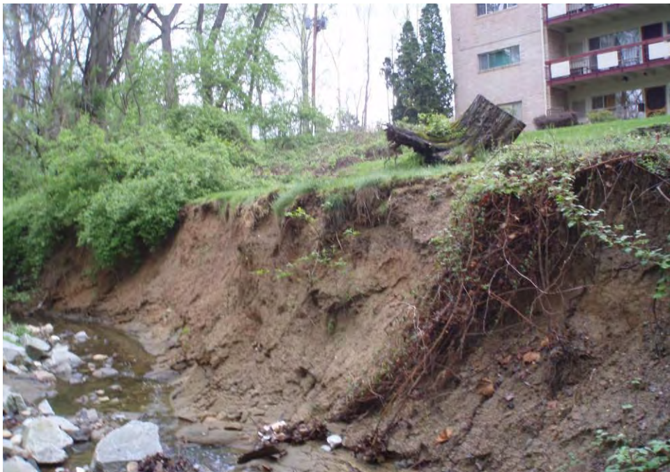
Site Photo: Incised channel with severe bank erosion in downstream portion of project
