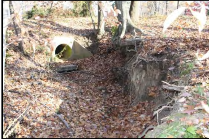
Figure 1: Severe meander bend erosion
