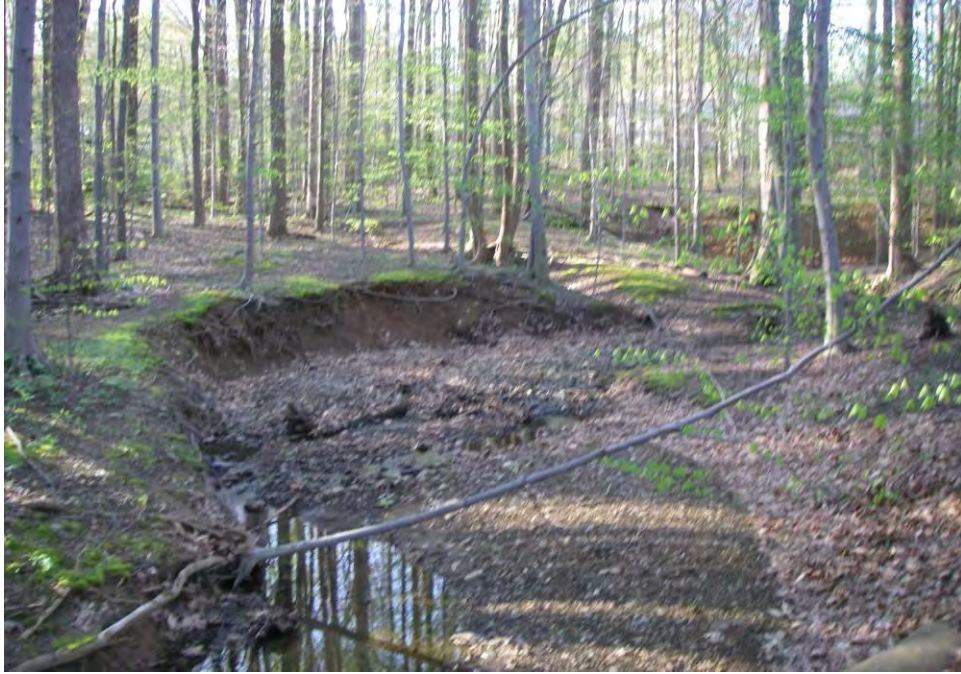
Site Photo: Over-widening channel with moderate to severe erosion
