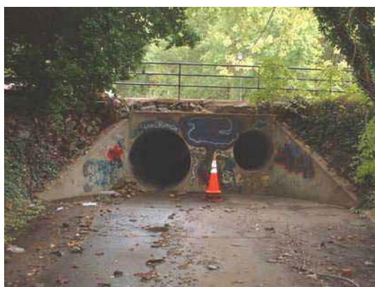
Photo 3.11 5' and 3' diameter pipes located under Linton Lane
