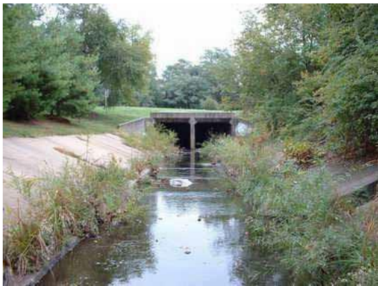
Photo 3.1 Double 8' x 8' outfall box culvert located under Fordson Road
