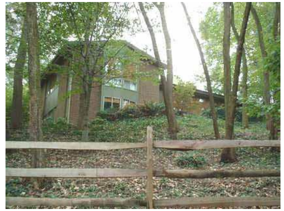
Photo 3.15 Deficient buffer zone along the tributary LHLH012 located on the west side of South Little Hunting Creek
