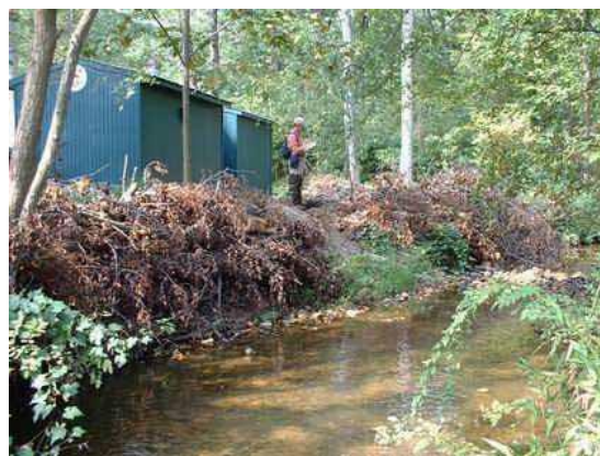
Photo 3.29 Deficient buffer area along the downstream segment of Paul Spring Branch north of Sherwood Hall Lane
