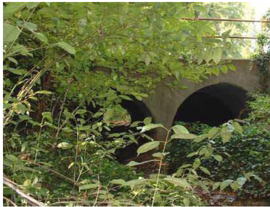
Photo 3.31 Double 72" corrugated metal pipe culverts located under Sherwood Hall Lane
