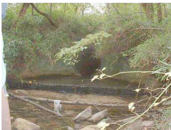
Photo 3.10 5' diameter concrete pipe located under Brady Street
