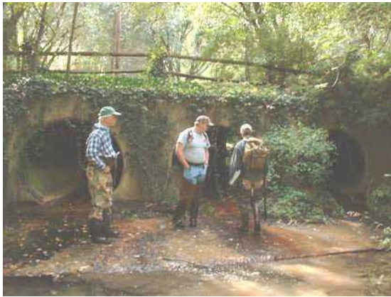
Photo 3.30 Triple 60" corrugated metal pipe culverts located under Davenport Street
