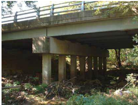
Photo 3.2 Sediment and debris causing a moderate impact downstream of Janna Lee Avenue bridge crossing
