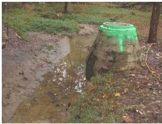
Photo 3.6 Raised manhole obstructing the flow of the tributary located north of Audubon Avenue
