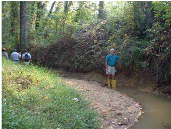
Photo 3.26 Severe erosion of 6' height was observed west of Admiral Drive
