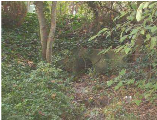
Photo 3.12 2' (diameter) concrete pipe located under Wessynton Way
