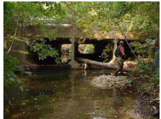
Photo 3.17 Four 10'x 6' concrete box culverts located under Sherwood Hall Lane
