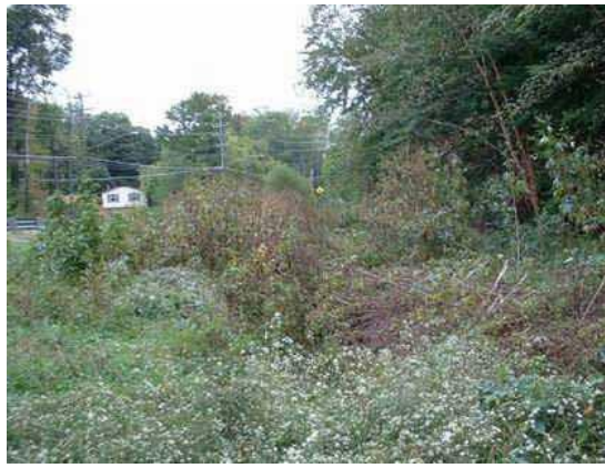
Photo 3.40 Buffer zone next to Collingwood Road on the eastern tributary to North Branch
