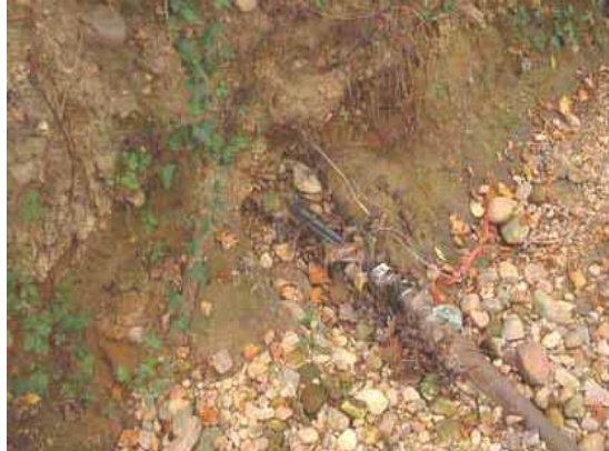
Photo 3.24 Partially buried telephone line south of the intersection of Rollins Drive and Radcliff Drive
