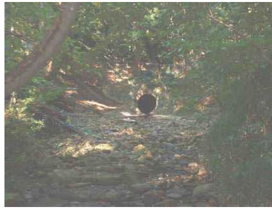
Photo 3.42 Concrete pipe outfall located west of Eaglebrook Court
