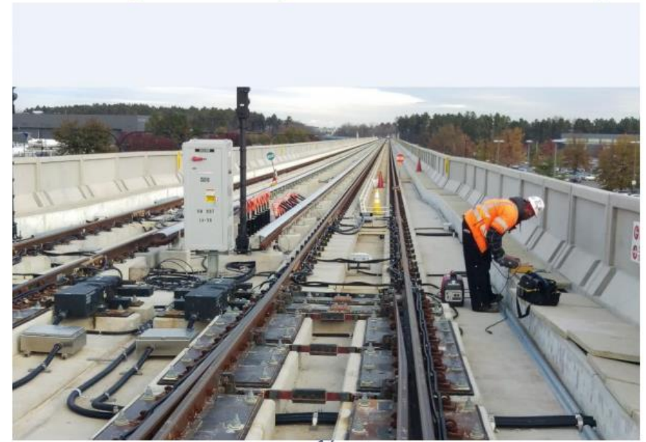
Installing Cable Trough Covers on Aerial Guideway
