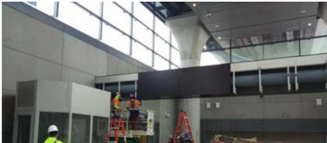
Installing Framing and Panels Over Gates at Dulles Station
