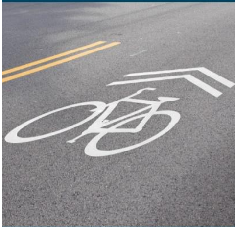
SHARED LANE MARKING (SHARROW)
