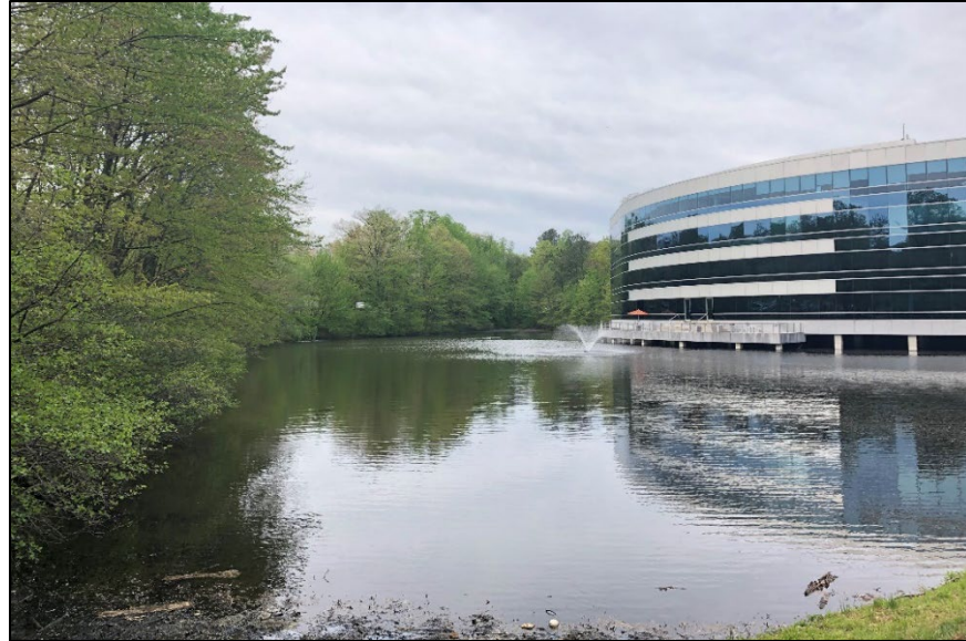
Figure 10. Stormwater Management Pond WP0323 (photo taken April 2019)
