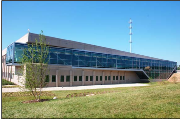
Construction is complete on the McConnell Public Safety and Transportation Operations Center (MPSTOC) facility.
