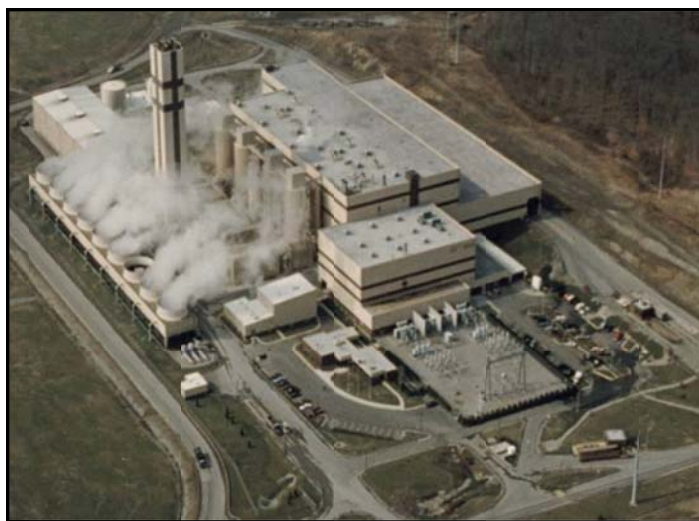
Aerial photo of the County's Energy Resource and Recovery Facility
