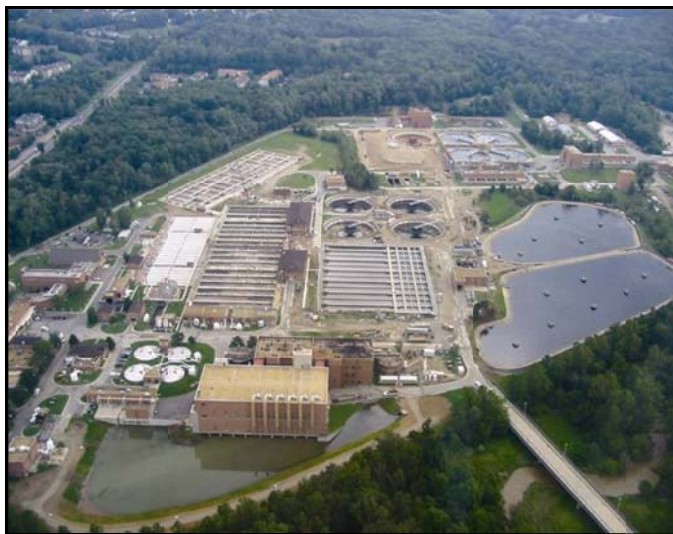
The County's wastewater treatment plant serves an estimated 364,500 households with public sewer service to help maintain a safe and caring community.
