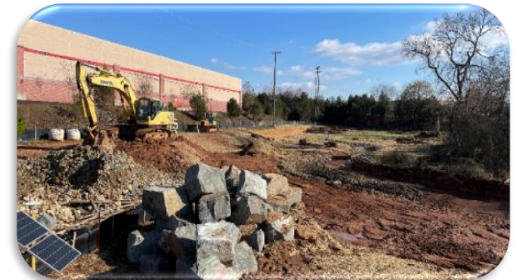
Schneider Branch Segment 1
