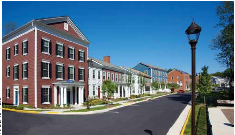
A base range of five unit types received layered treatments of a variety of materials, details, and colors to achieve a varied streetscape. Simplifying the unit types significantly reduced construction costs.
