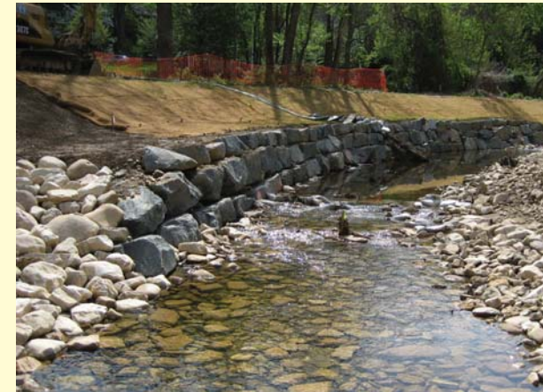
A recent stream restoration at Little Pimmit Run will improve stream water quality and stabilize the catastrophic erosion that was occurring. It cost over $500 a linear foot, but could be undermined by poor maintenance, cutting down the riparian buffer or an increase in impervious surface in the watershed.
