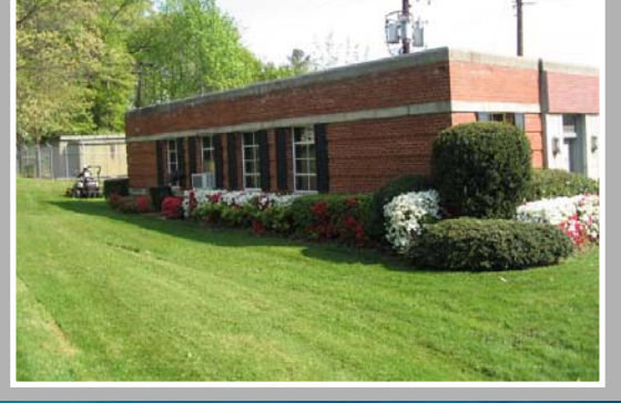
CHESTERBROOK PUMP STATION
