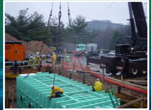
SCOTTS RUN PUMP STATION CONSTRUCTION
