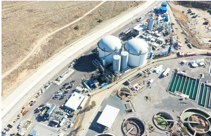
Figure 16: Anaergia's Rialto Bioenergy Facility (Largest Food Waste AD and Supplier of RNG Derived from Landfill Diverted Organics in North America)
