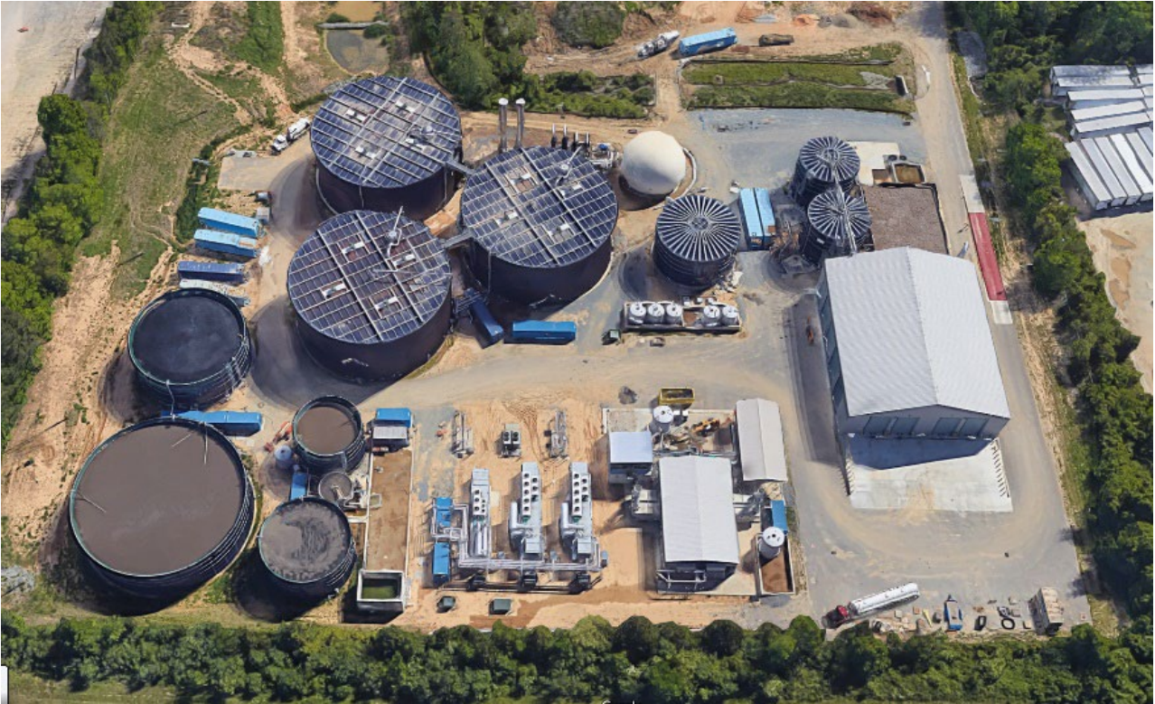
Existing Charlotte Bioenergy Facility
