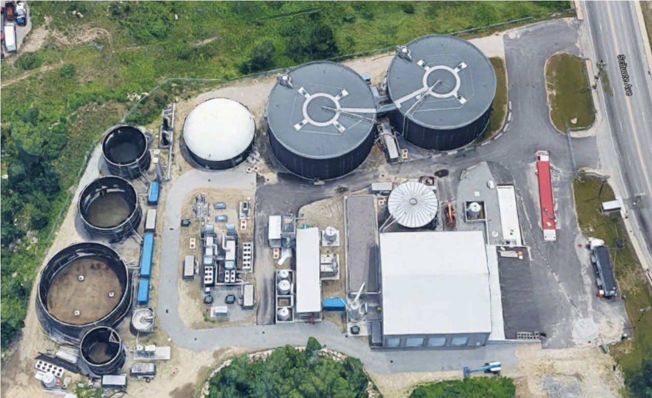
Existing Rhode Island Bioenergy Facility
