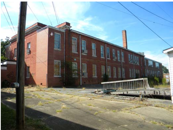
East Façade, Old School, Camera Facing Northwest
