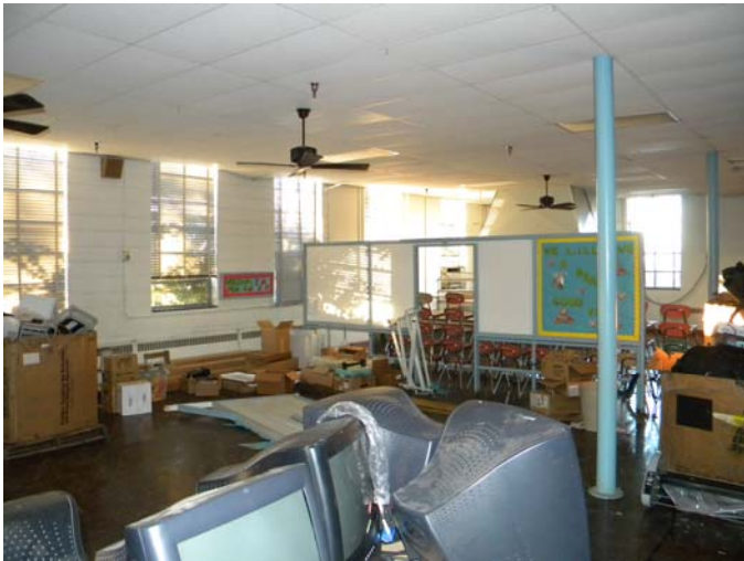
Cafeteria, 1952 Addition, Camera Facing Northwest
