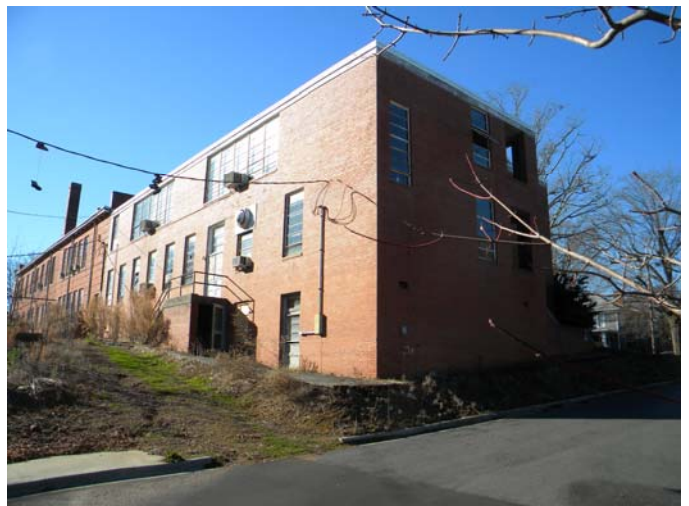
East Façade, Old School, Camera Facing Southwest
