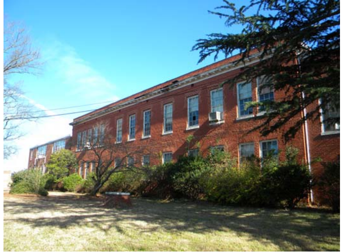
West Façade, Old School, Camera Facing Northeast
