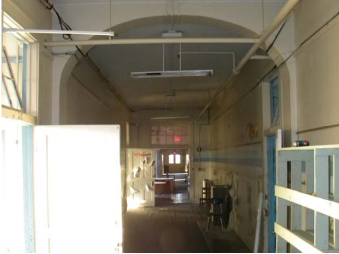
Main Corridor View, Old School, Camera Facing North
