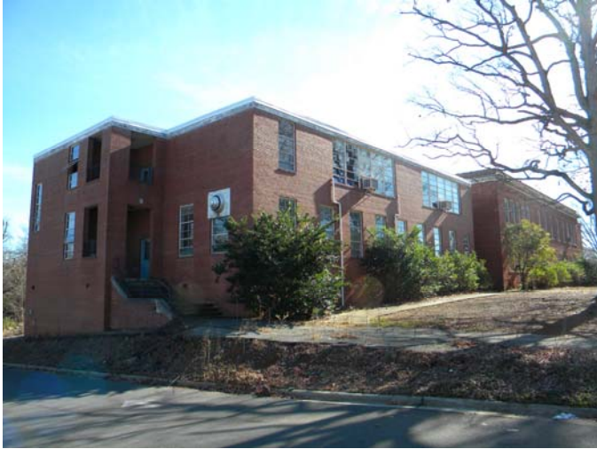
West Façade, Old School, Camera Facing Southeast
