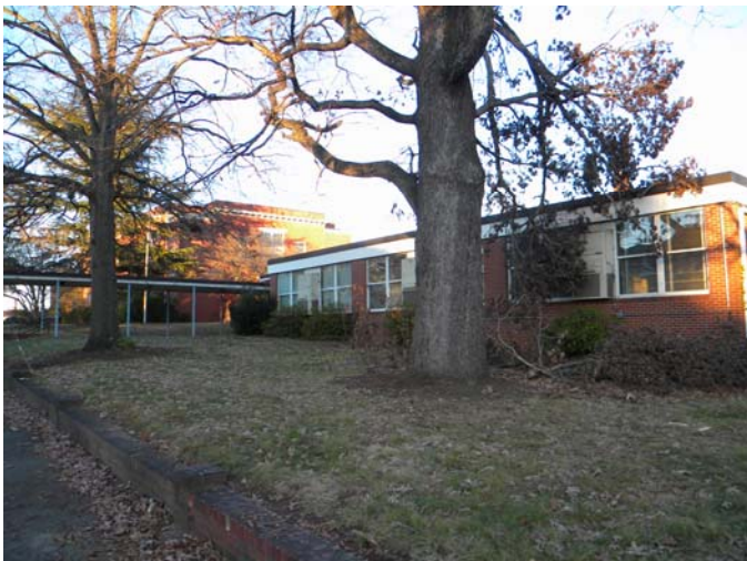
West Façade, 1965 School, Camera Facing Northeast
