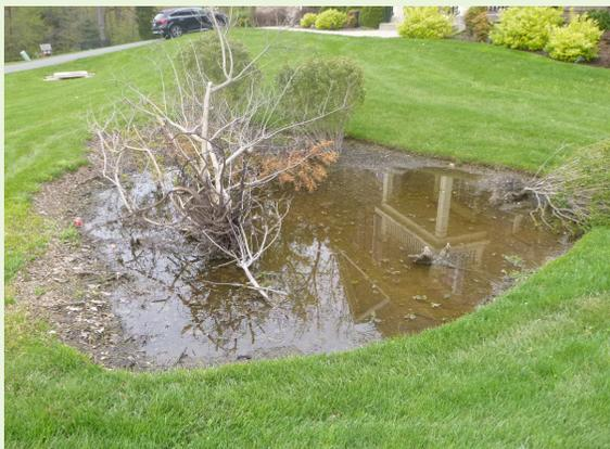
Photo 3 - Ponding water in the facility for more than 48 hours.
