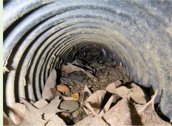
Photo 2 - Inflow pipe blocked by debris and sediment.
