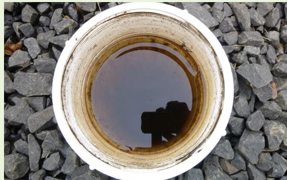
Photo 4 - Standing water observed inside observation well for more than 48 hours.
