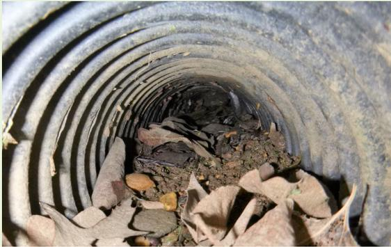
Photo 1 - Inflow pipe blocked by debris and sediment.
