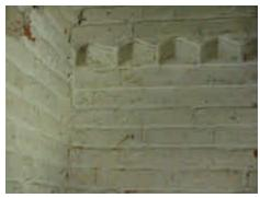
present wooden cornice, indicating, along with the fact that brick bonding continues into the gable end, that the roof configuration on the wings is probably original. The only probable differences between the original roof and what is now in place is that the gable ends over the center section were clipped, giving the appearance of a hip roof when seen from the front. This roof continued, shed style, over the wings.
