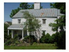
This structure reportedly burned in 1947 leaving only the exterior brick walls. However, there is no burn evidence in the attic or from archaeological excavations adjacent to the structure. The windows, doors and interior features are modern, but whether this is due to a fire or done to update
