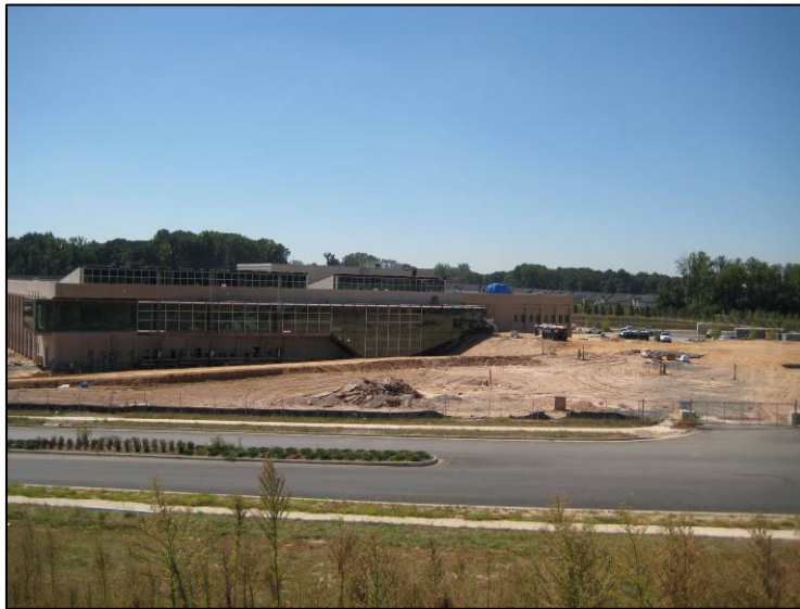
Construction is well underway on the Public Safety and Transportation Operations Center (PSTOC) facility.
