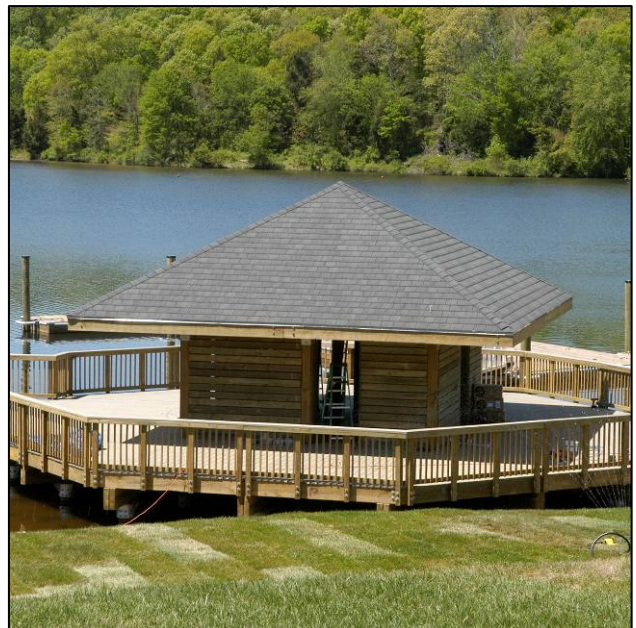
Picture of new dock at Lake Fairfax.
