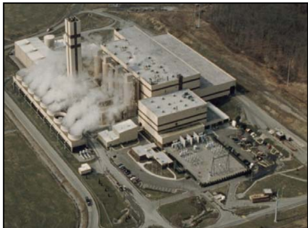
I-95 Energy/Resource Recovery Facility
