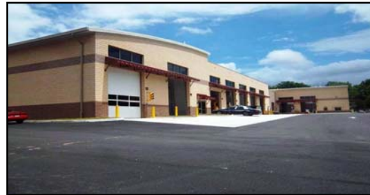
Renovation and expansion at the Newington DVS Facility in Mount Vernon District
