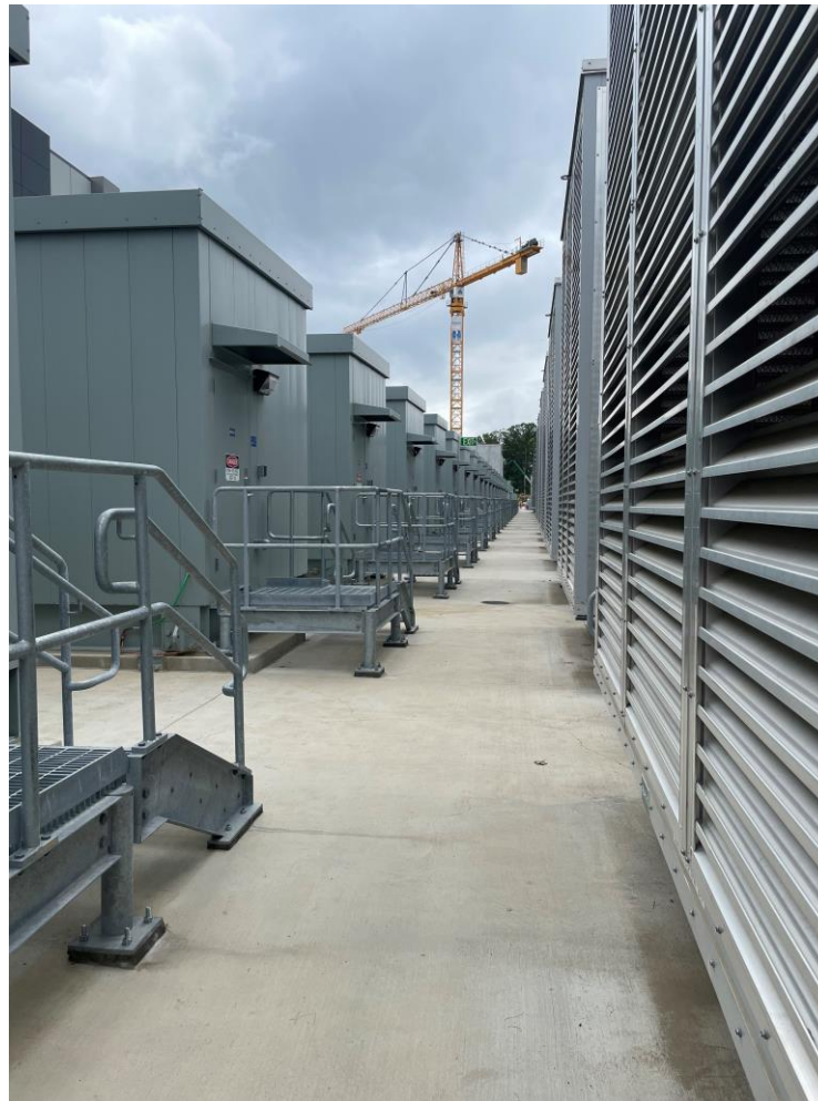
Generators (outside and inside enclosure), Stack Infrastructure, Manassas
