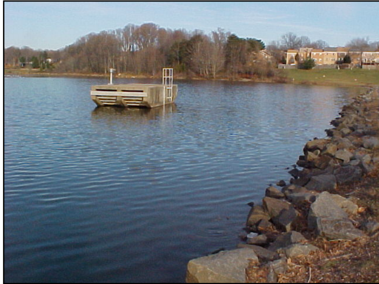
Photo of Lake Royal which is part of the County's extensive stormwater system that includes 1,800 miles of storm drainage conveyance systems, 45,000 stormwater drainage structures, and 1,104 stormwater management ponds.
