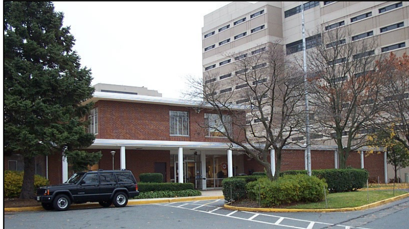
Photo of the Police Annex Building in Fairfax City, built in 1960, which is one of many aging buildings within Fairfax County.
