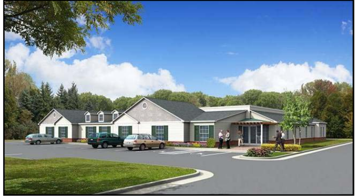
Artist rendering of the Gregory Drive Facility to accommodate the therapeutic mental health and substance abuse program for County residents.
