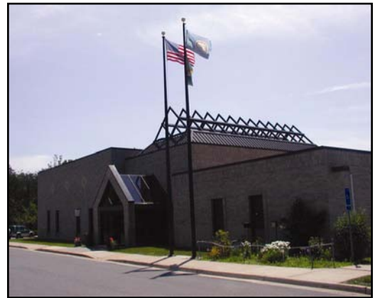
Photo of the Mott Community Center.
