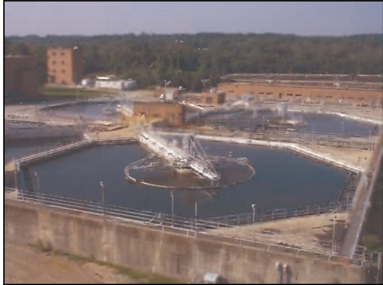
Photo of the Noman M. Cole Jr. Pollution Control Plant
