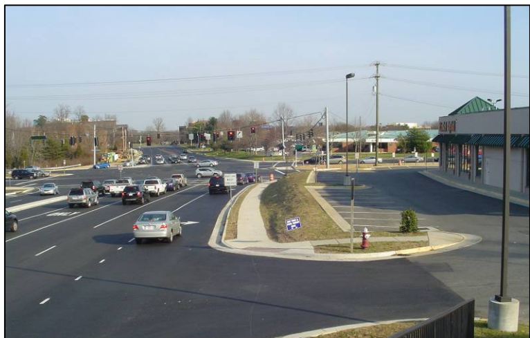
Picture of Route 50/Waples Mill Road.
