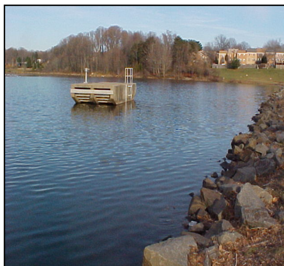
Photo of Lake Royal which is part of the County's extensive stormwater system.
