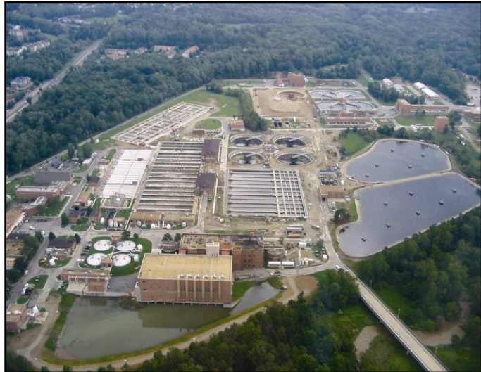
The County's wastewater treatment plant serves an estimated 362,375 households with public sewer service to help maintain a safe and caring community.
