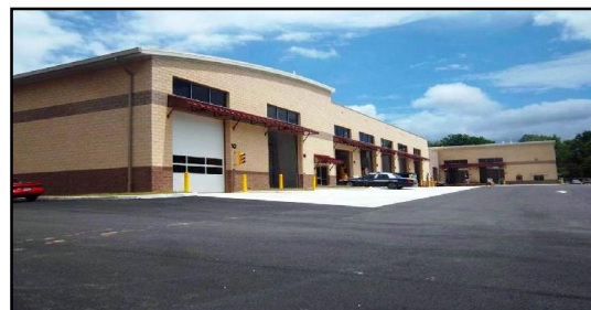
Renovation and expansion at the Newington DVS Facility in Mount Vernon District
