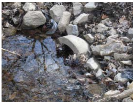
Existing pipes in failure condition
