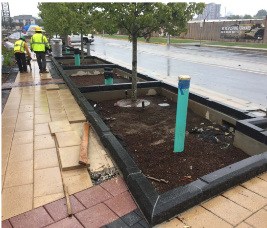
Capital One Under Construction
