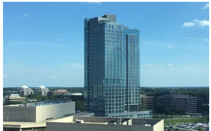
Lumen, Tysons' newest residential building
