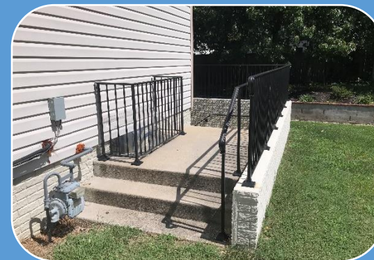
Modified basement areaways
