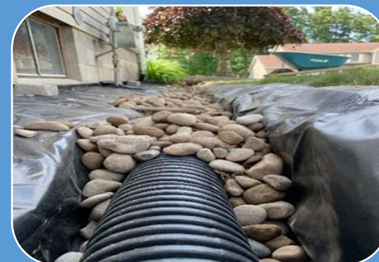
Exterior grading or drains
