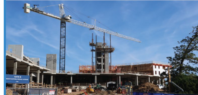
Ovation at Arrowbrook 274 Multifamily Units Dranesville District
