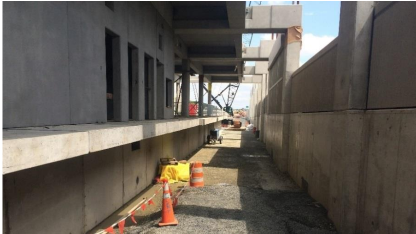
Unfinished platform and interior station wall
