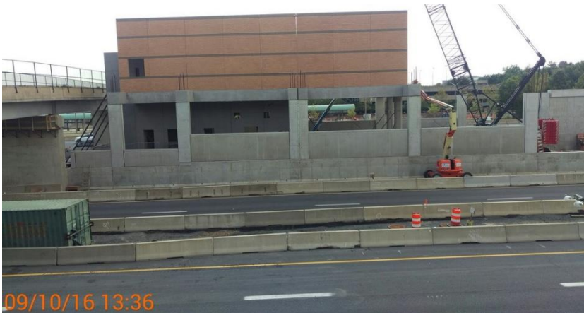
Station Wall Panels and Exterior
