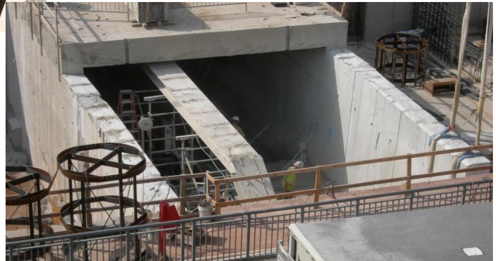
Pedestrian Tunnel to Terminal
