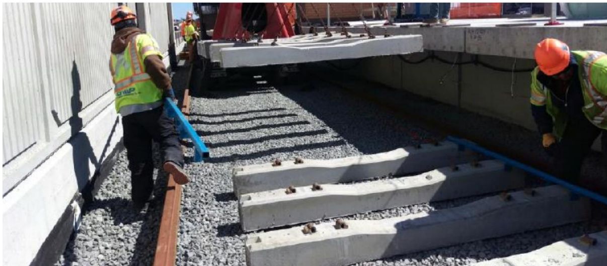
Set Concrete Ties and Rail for Innovation Station Outbound Track
