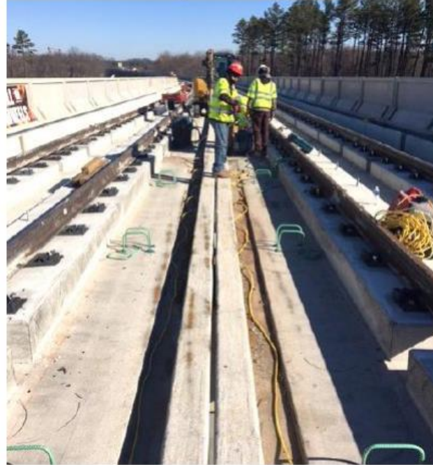
Prepare for Concrete Pours and Set Rails on Elevated Guideway
