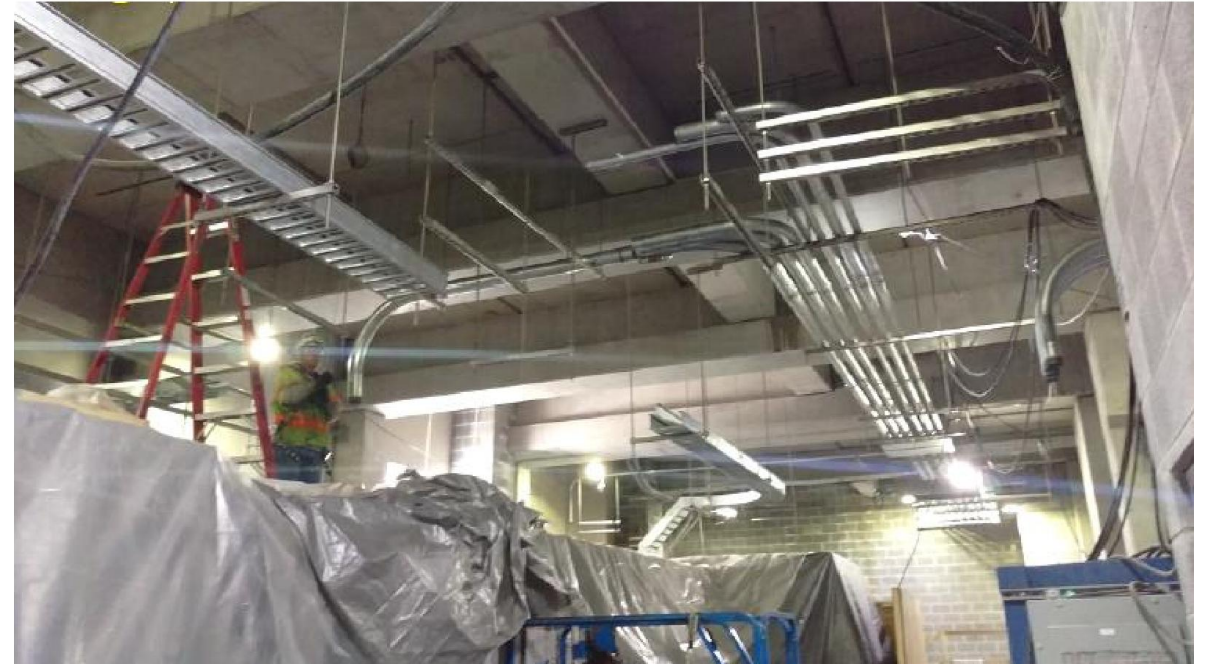
Install Overhead Conduits and Feeders to AC Switch Gear in Dulles Station
