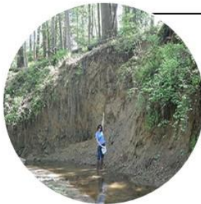
Erosion along Difficult Run
