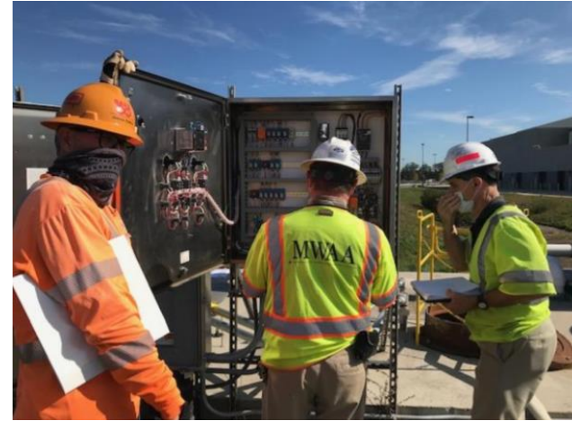
Sanitation Lift Inspection at the Yard
