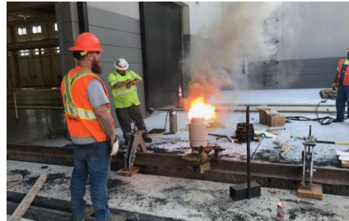
Thermite Welding Replacement Insulated Joint 'Plug' in Place
