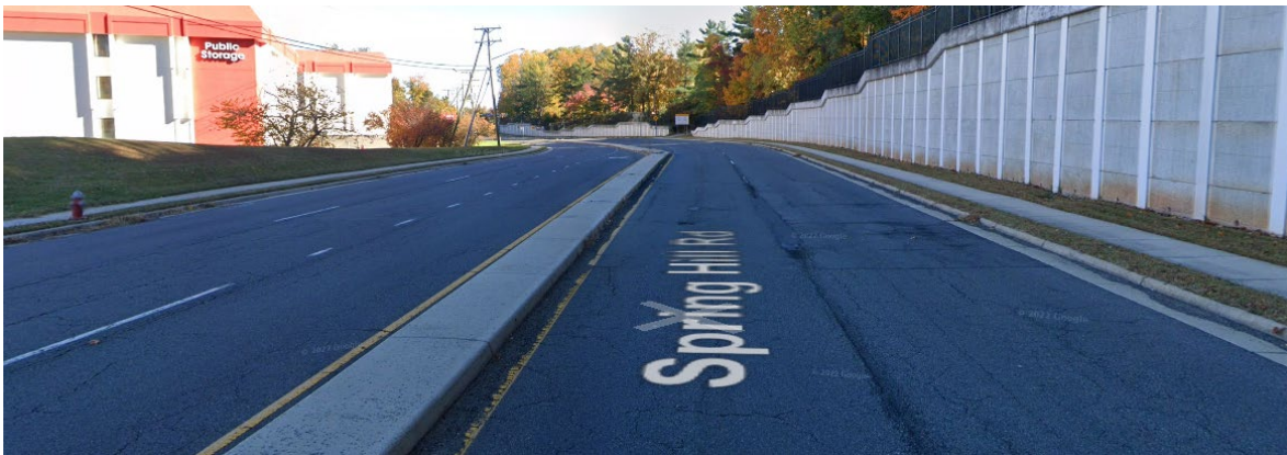
Figure 6: Spring Hill Road (four lanes), eastbound to International Drive
