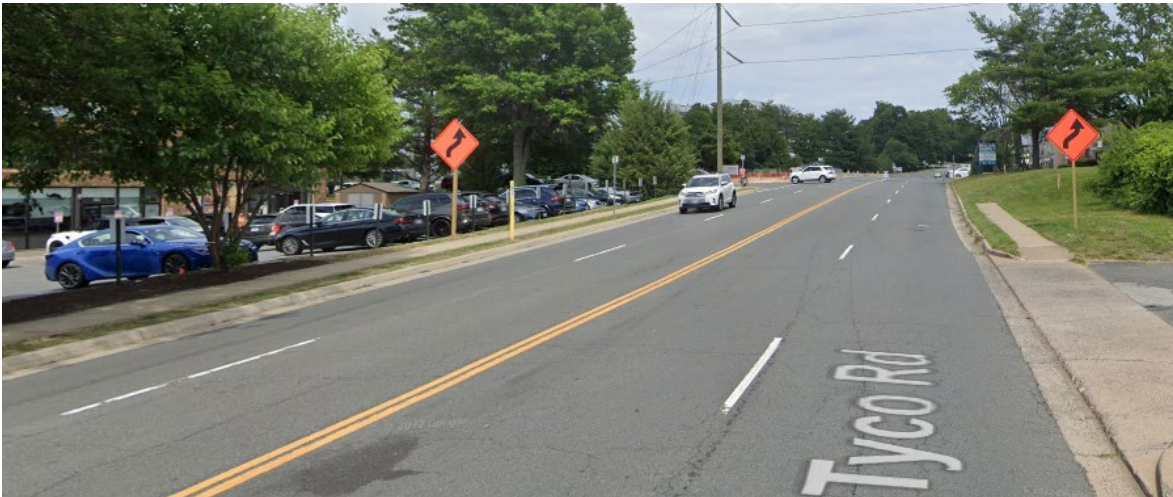
Figure 7: Tyco Road (four lanes), eastbound to Spring Hill Road
